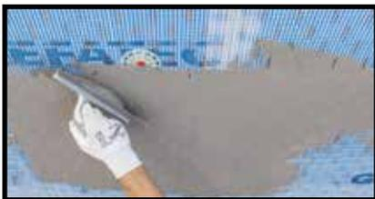
Smooth and fill the mesh with a notched trowel in a vertical direction
