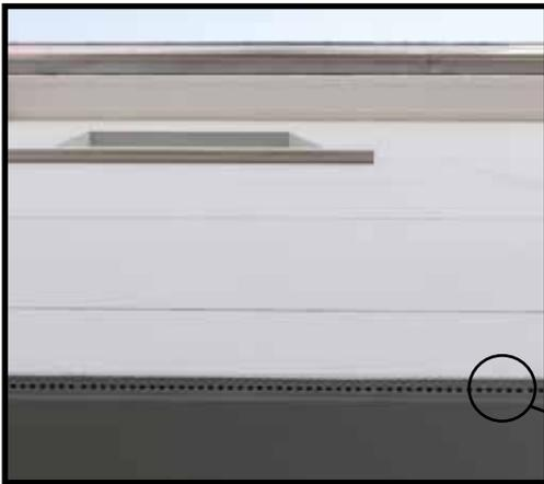
The special, patented CeraVent® matting **CeraVent®** favours drainage, ventilation and decoupling.
