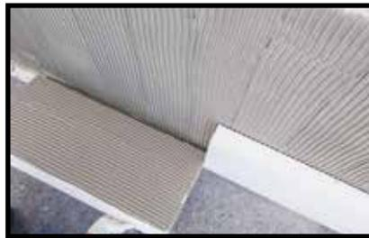
Installation of insulation panels with double buttering
